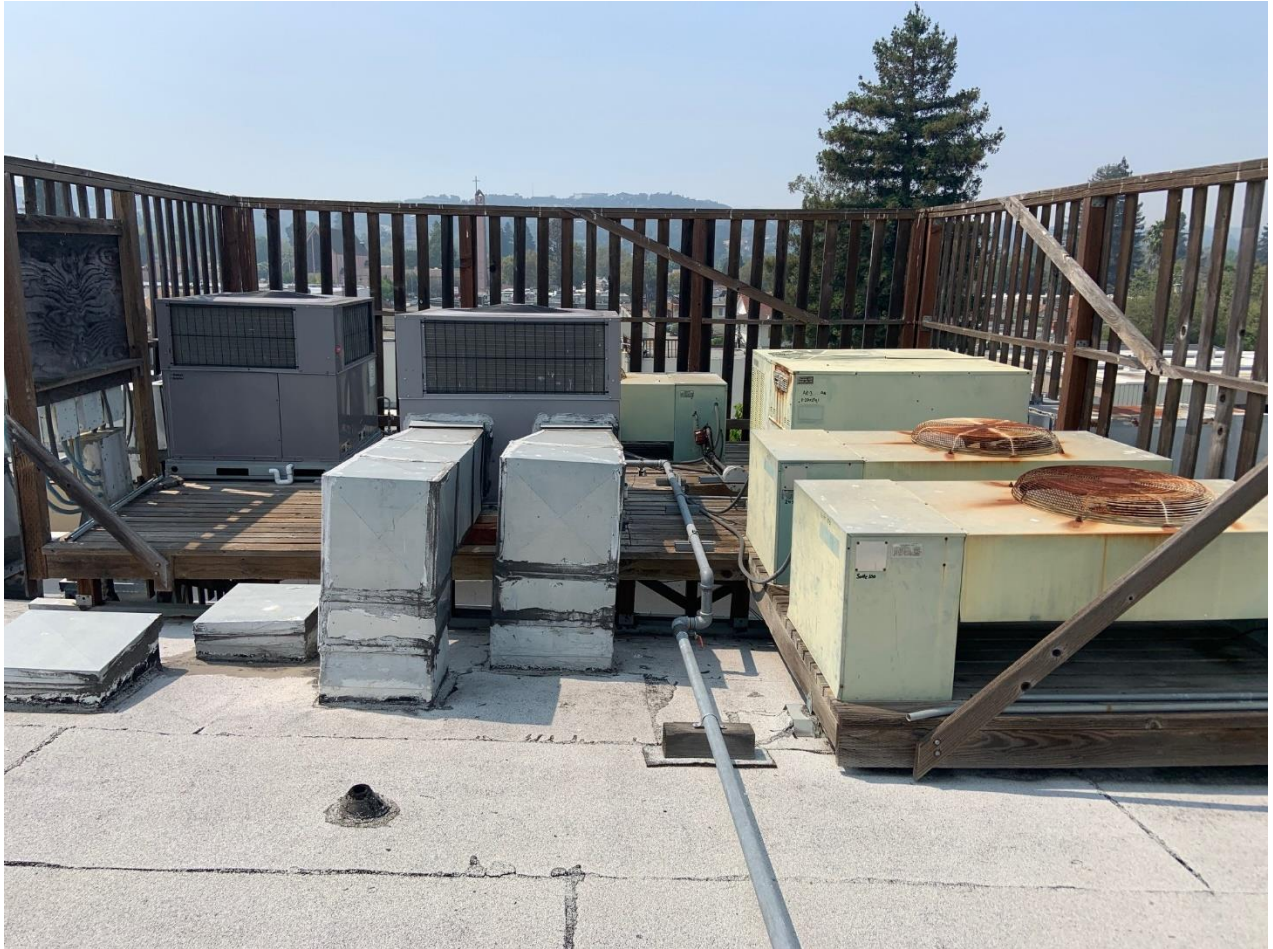
Existing Roof Deck
